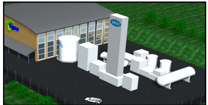
Fig. 2: Schematic view of the Air Separation Unit (ASU) adjacent to the main P&D Plant building.
