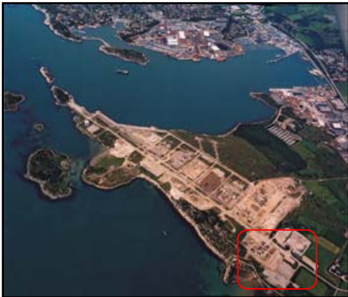
Fig. 1: Aerial view of reclaimed land area at the Energy Park, Risavika, nr. Stavanger, South Norway. Highlighted rectangle shows proposed location for the P&D Plant.
