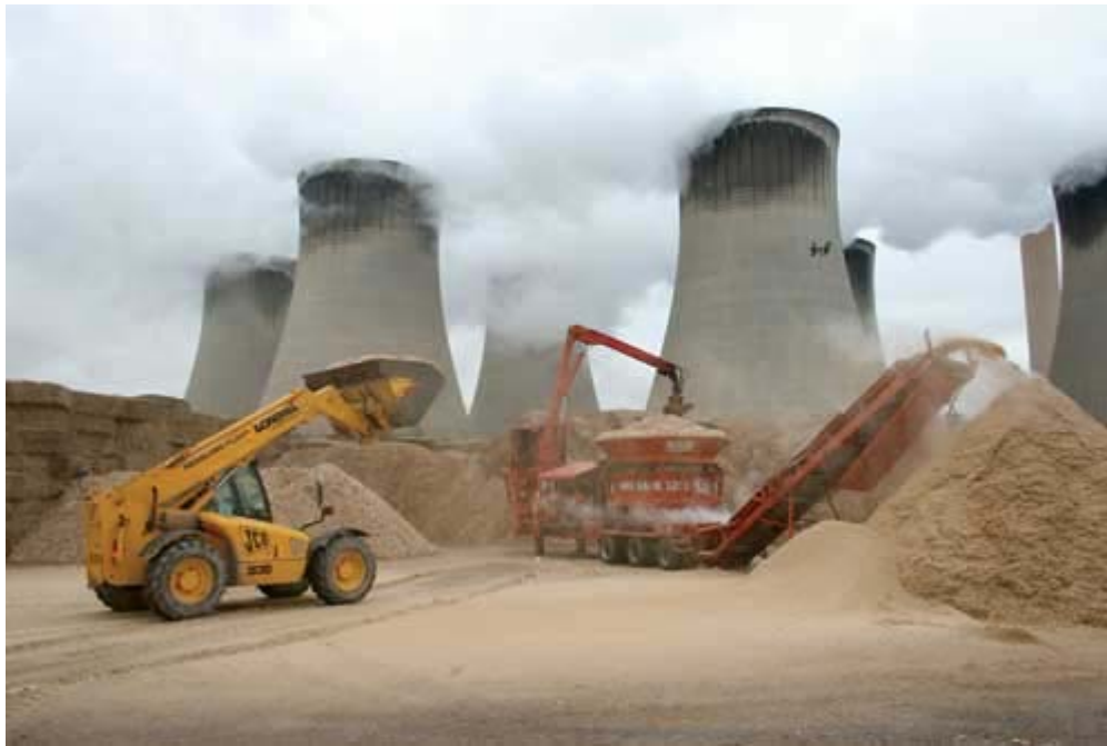
The 4 GW Drax Power Station in North Yorkshire, England, is one of the largest biomass co-firing facilities in the world. Here the biomass is being processed prior to combustion.
